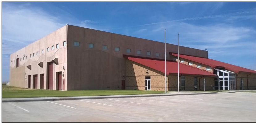
The 15 mgd South Water Treatment Plant in Lubbock, Tex., came on line in 2012. Photo courtesy of the City of Lubbock, Tex.
