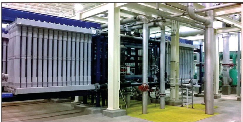
The South Water Treatment Plant has six individual microfiltration skids, each with a 2.5 mgd filtration capacity. Photo courtesy of the City of Lubbock, Tex.
